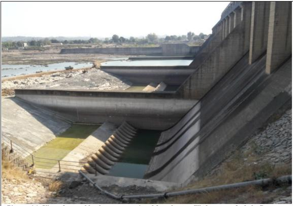
Picture 6.1: View of treated bucket segments 1 and 2, and water filled segment 3 of the Bansagar dam
